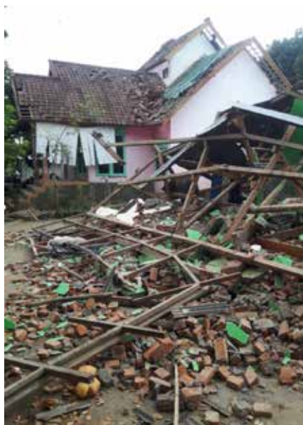
A home destroyed in North Lombok.
